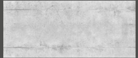
Flat E Betonwand
